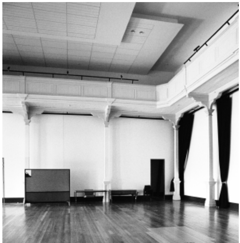
29 The central part of the exhibition hall after recent conversion work. The space beneath the central void in the mezzanine has been enclosed with walls below the mezzanine and with a ceiling above.
